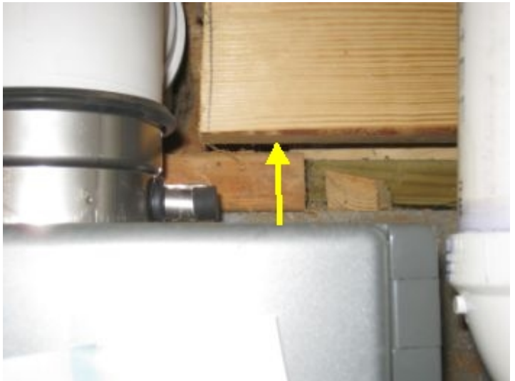
Improper clearance to combustibles at water heater
