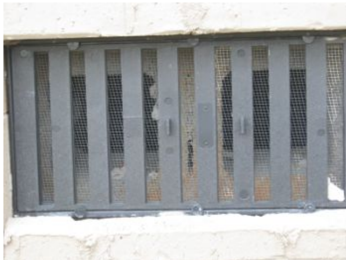
Correctly installed foundation vent
