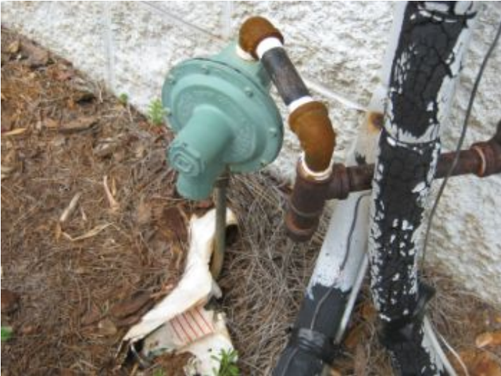
Properly replace gas lines as needed for function and safety Unprotected gas line - Exterior gas lines should be protected from physical damage to reduce risk of leakage. Correct as needed for safety.
