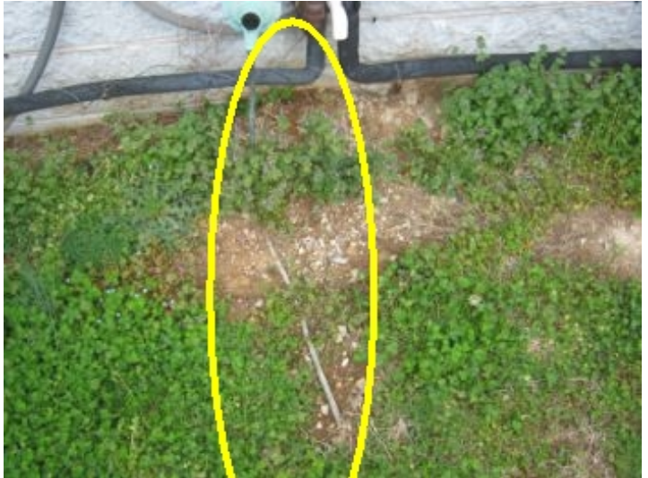
Properly replace gas lines as needed for function and safety Unprotected gas line - Exterior gas lines should be protected from physical damage to reduce risk of leakage. Correct as needed for safety.
