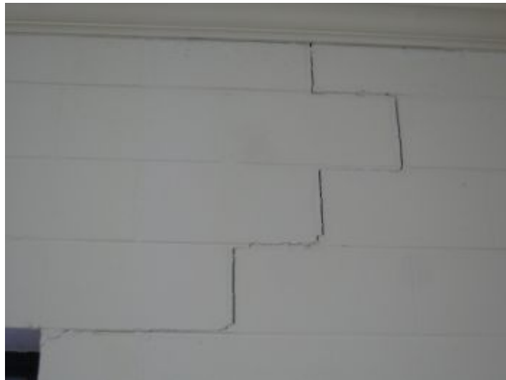
Monitor settlement cracks
